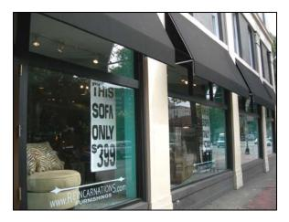
Awnings and canopies should be made of treated, weather-durable fabric such as canvas or woven acrylic. Vinyl, metal, and plastic are not appropriate awning or canopy materials.
